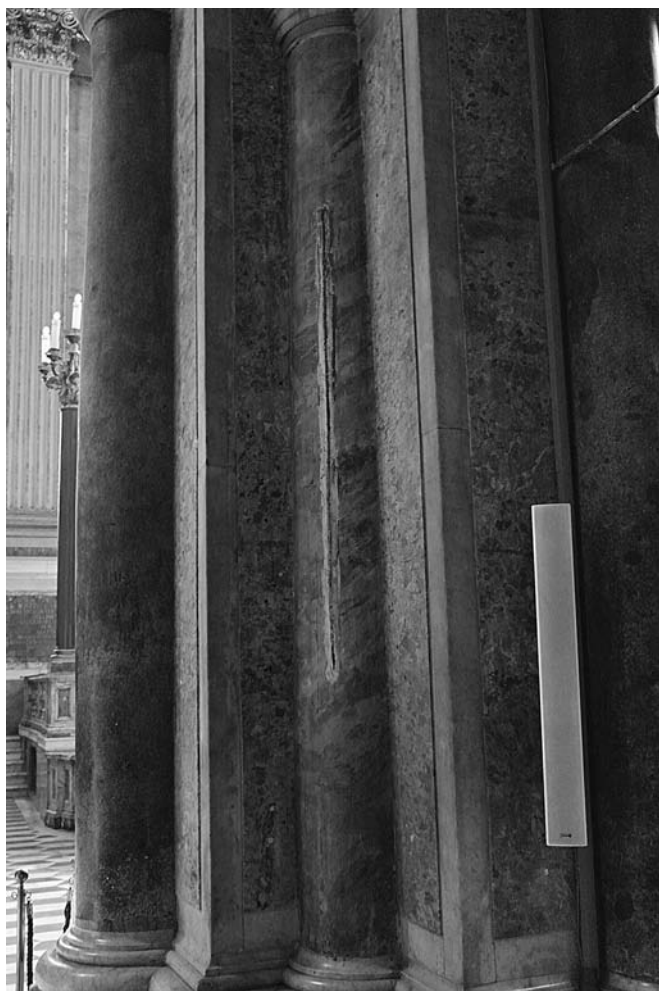
3.5 | The seven-palm canna plastered in a pier of Naples Cathedral. Photograph by the author.
