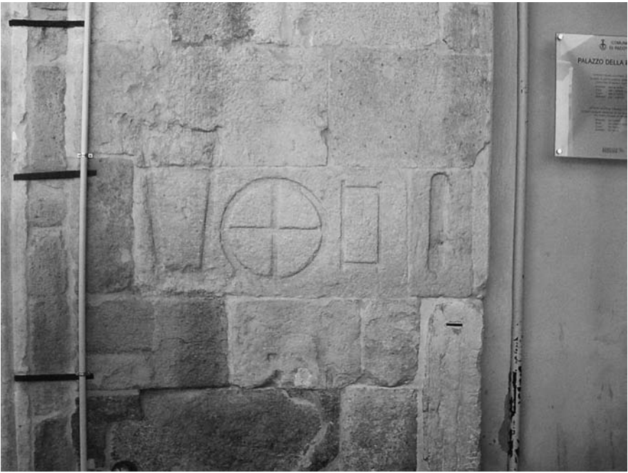
12.2 | The measurement standards on Padua's Palazzo della Ragione, near the staircase of the birds ( oseri ): the roof tile (left), the crossed bread shape (center), and the brick (right). At the bottom right, the metal plaque marks the upper end of a broken length standard, either the brazzolaro (the length for cloth) or the pie de di fabbrica . Photograph by the author.
